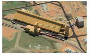
Potash and Salt Compaction Facility Basic engineering design for a facility that was designed to produce 680,000 TPY of food grade fine bagged salt, food grade bulk salt, water softener packaged salt, extra course packaged salt, road salt and agriculturally enriched blocks. The facility also produced 533,000 TPY of granular potash.
